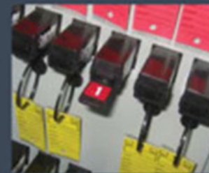
Access key remains while the keys are checked out
